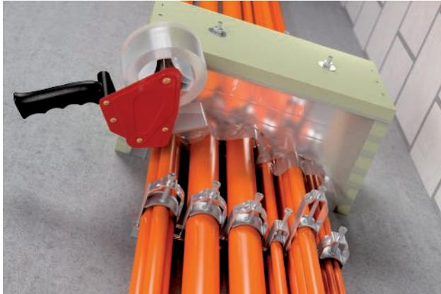
Creating a casing for the secure filling of the housing
