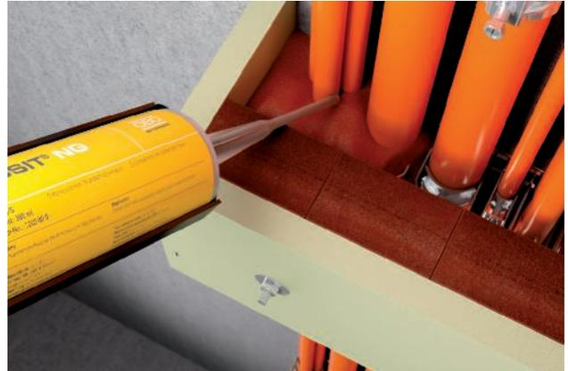
Filling with PYROPLUG® Block foam block and filling the gaps between cables with the PYROSIT® NG fire protection foam
