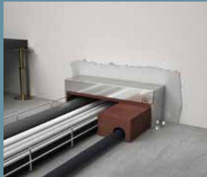
Insert the cut inlay block into the larger cavities
