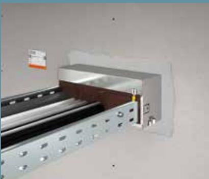
Connect the equipotential and apply the identification plate
