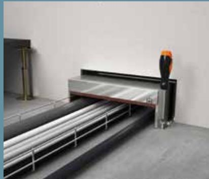
Insert the box into the wall opening and fasten in the base
