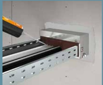
Completely close the cavities with PYROSIT® NG fire protection foam
