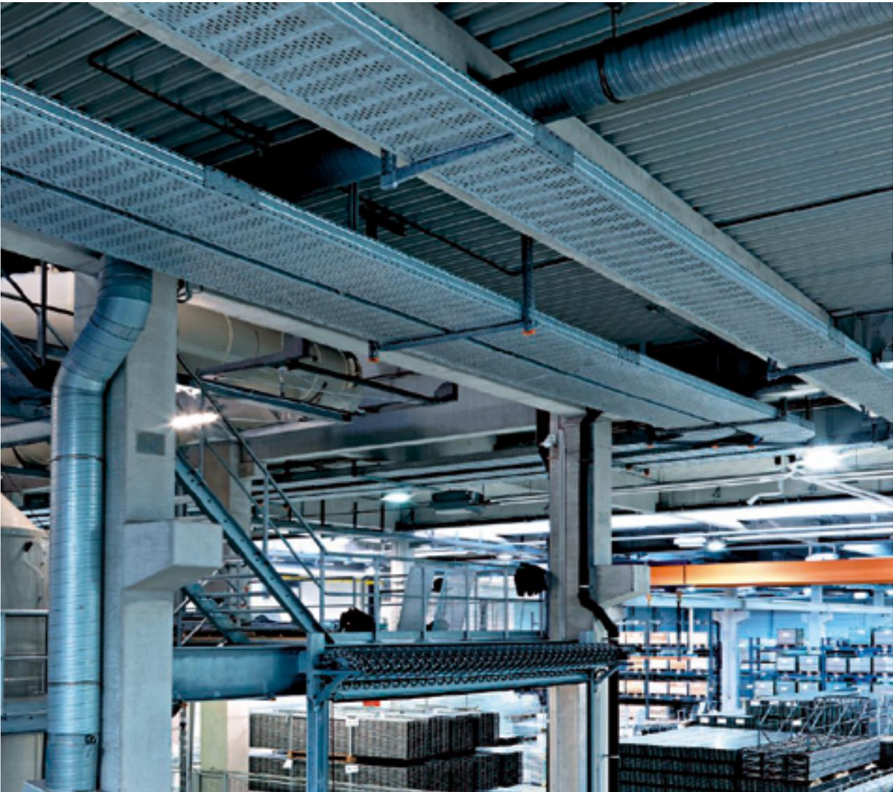
When you need to bridge wide spans and support high cable loads, the OBO wide span cable trays are the perfect solution. The product range comprises cable trays with widths of between 200 and 600 mm and side heights of 110 to 160 mm. Comprehensive system accessories, such as fittings and all the fastening materials for concrete and steel mounting, round off this product range perfectly. OBO wide span cable trays have proven their
